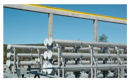
Ultrafiltration membrane bioreactor (MBR)
